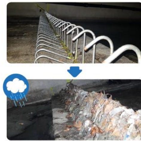
Solid waste retention systems in combined sewer overflow points
